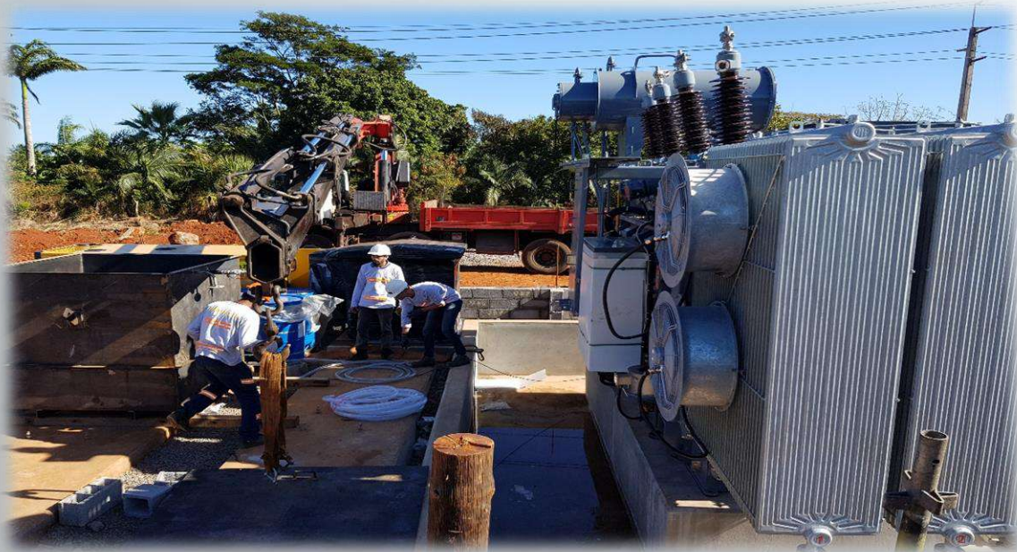
Transportation and Fixing of 22/66KV TX
